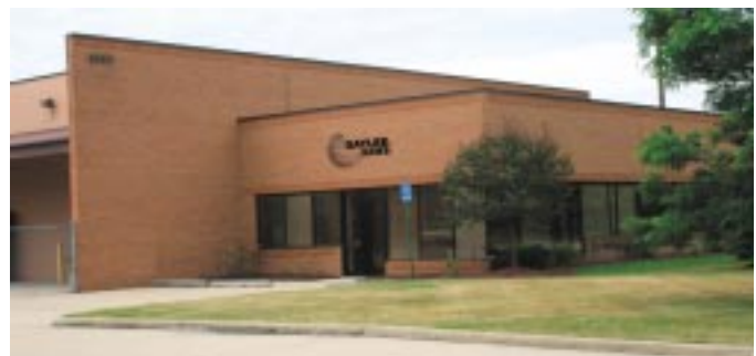
Gaylee's modern manufacturing facility located in Sterling Heights, Michigan.
