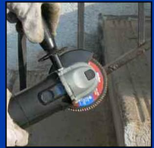
Removing rust from a railing before painting.
