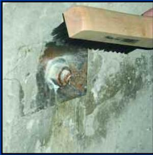
Removing excess concrete from the surface of a steel support plate.
