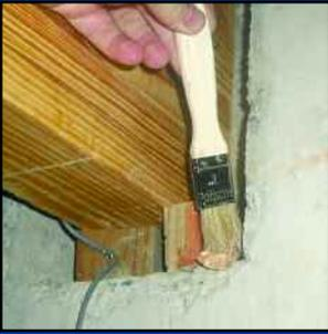
Clearing debris from a crevice with a chip & oil brush.
