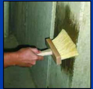
Applying waterproofing material with a masonry brush.
